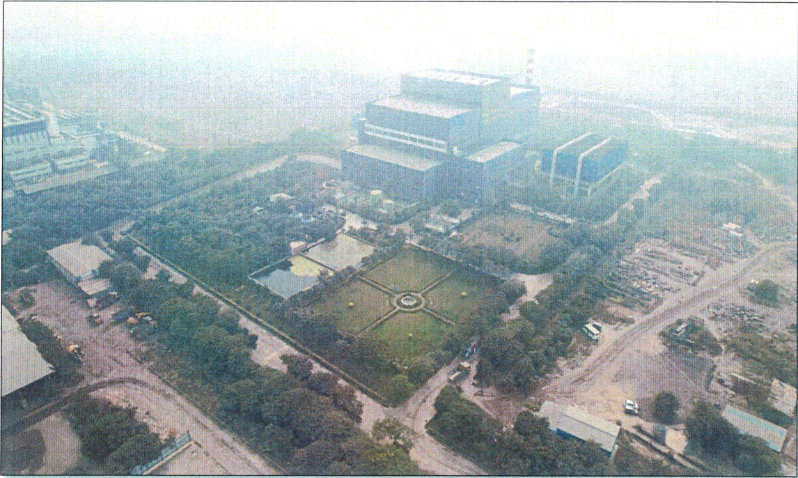
Fig: 2x600 TPD RDF based power Plant at Bawana, Delhi
