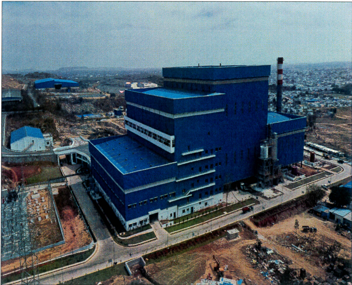
Fig: 2x600 TPD RDF based power Plant at Jawaharnagar, Hyderabad
